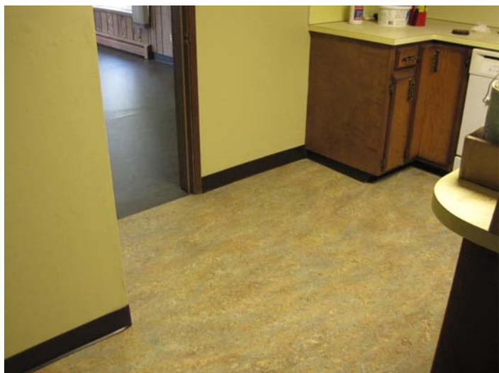
New Forbo marmoleum floors were installed in the multipurpose room and in the kitchen. Existing hardwood floors were refinished in the large office, and new hard surface floors will be installed in the two smaller offices.
