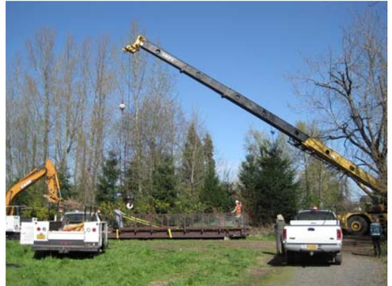
Several cranes were required to move the heavy bridge to its permanent location at Whitaker Ponds.
